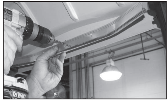
Figure 5 - Rear Track Installation
